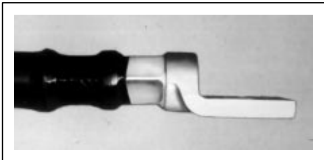
FIG. 22. COMPLETED POWER CABLE TERMINAL. E-16355.
